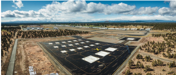
New heliport at the Bend Airport
